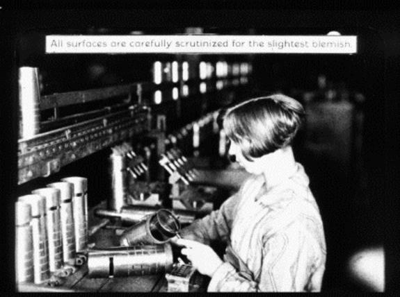
Diameter, length, thickness and alignment all come in for their share of attention. Edges of ports, oil arooves, holes and slots, alignment, size and finish of sleeve rod lug and bevel of the ends are all carefully examined, and checked against specifications before -
