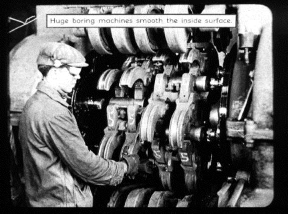
Following this first rough boring operation the sleeve is inspected and tested for proper diameter and passed to --
